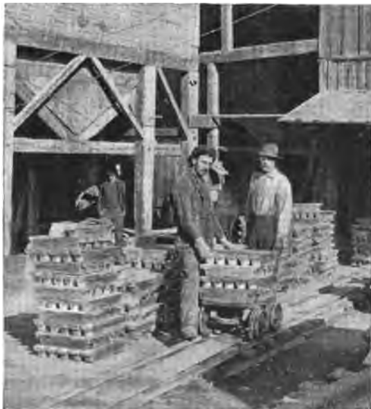
BULLION AT THE AMERICAN SMELTER, LEADVILLE, COLORADO
