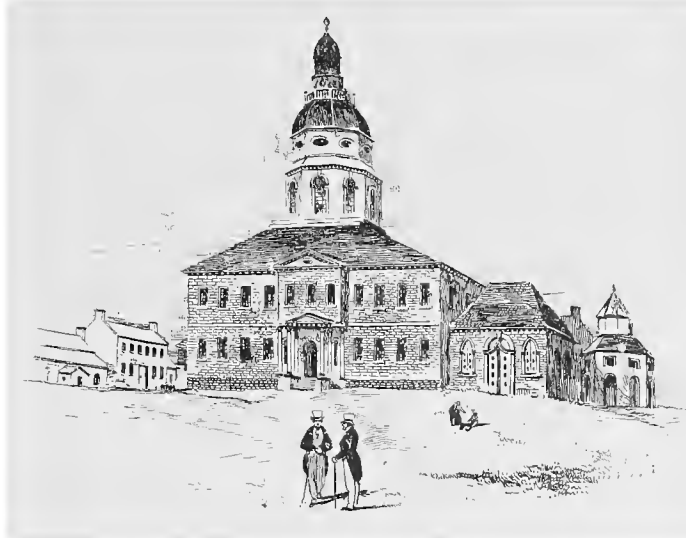
OLD STATE HOUSE AT ANNAPOLIS, MARYLAND
