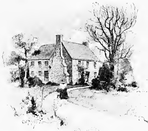
HOUSE AT GUILFORD, 1639
