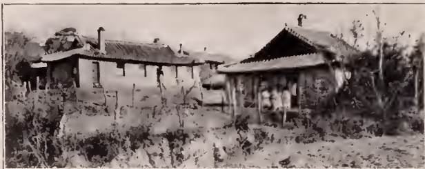
Kunsan Hospital Buildings.
