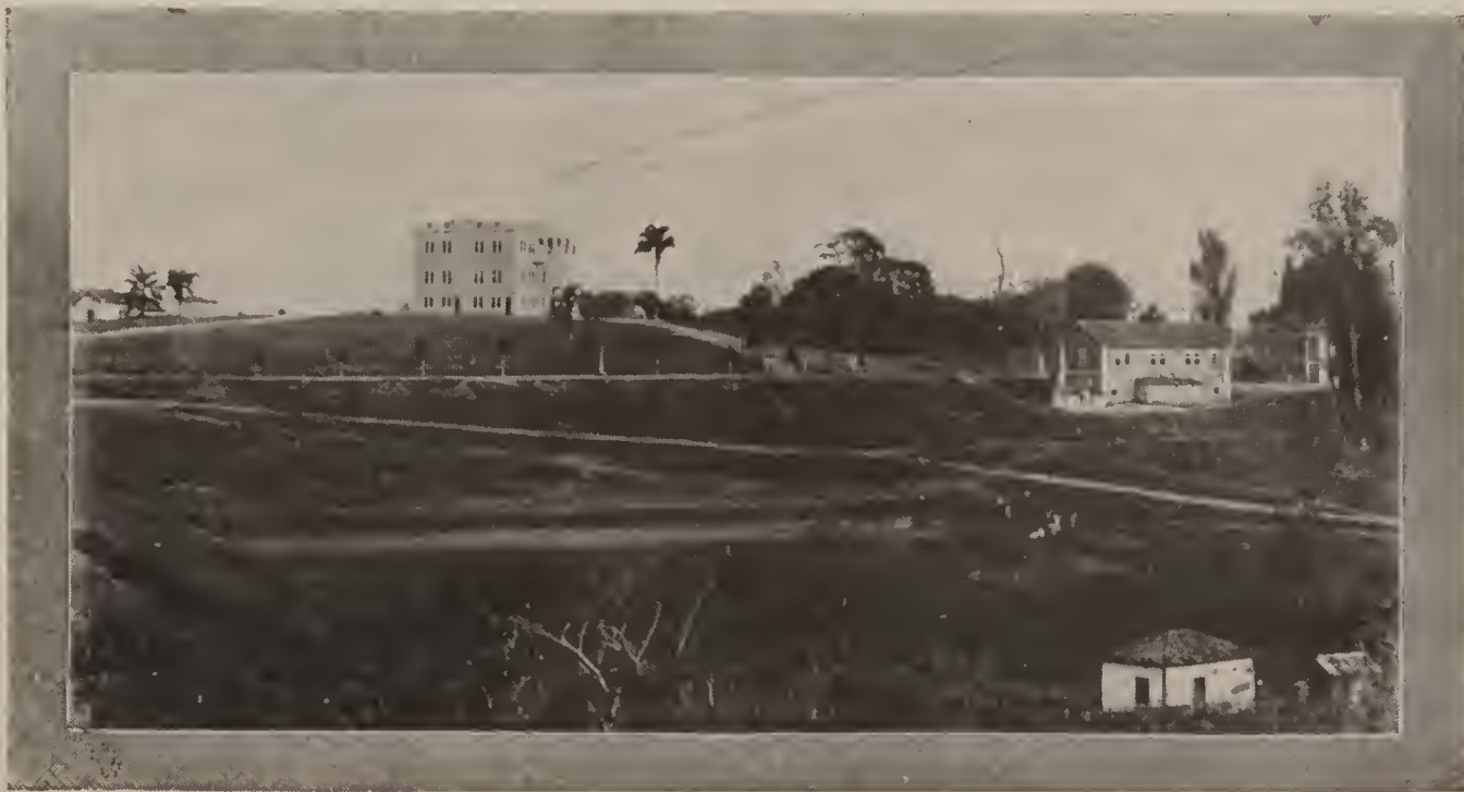
LAVRAS SCHOOL BUILDINGS, BRAZIL.
