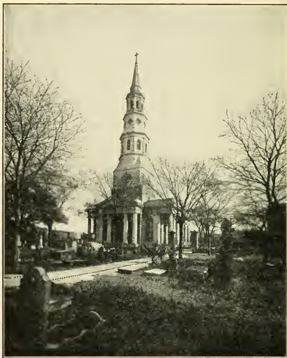
ST. PHILIP'S CHURCH, CHARLESTON
