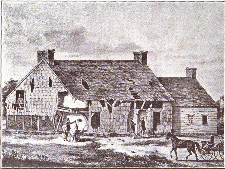
OLD TENNENT PARSONAGE, BUILT 1706
