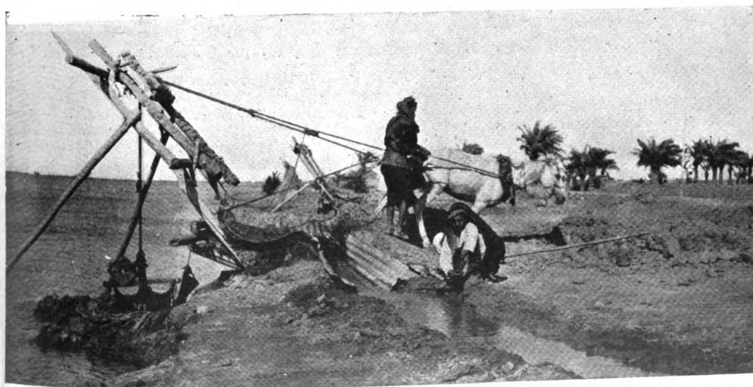
Method of Irrigating as practiced in Mesopotamia.
