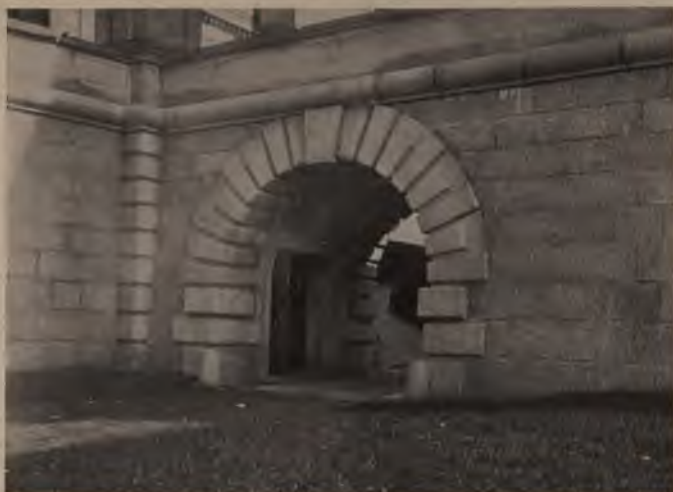
THE SOUTH ARCHWAY
