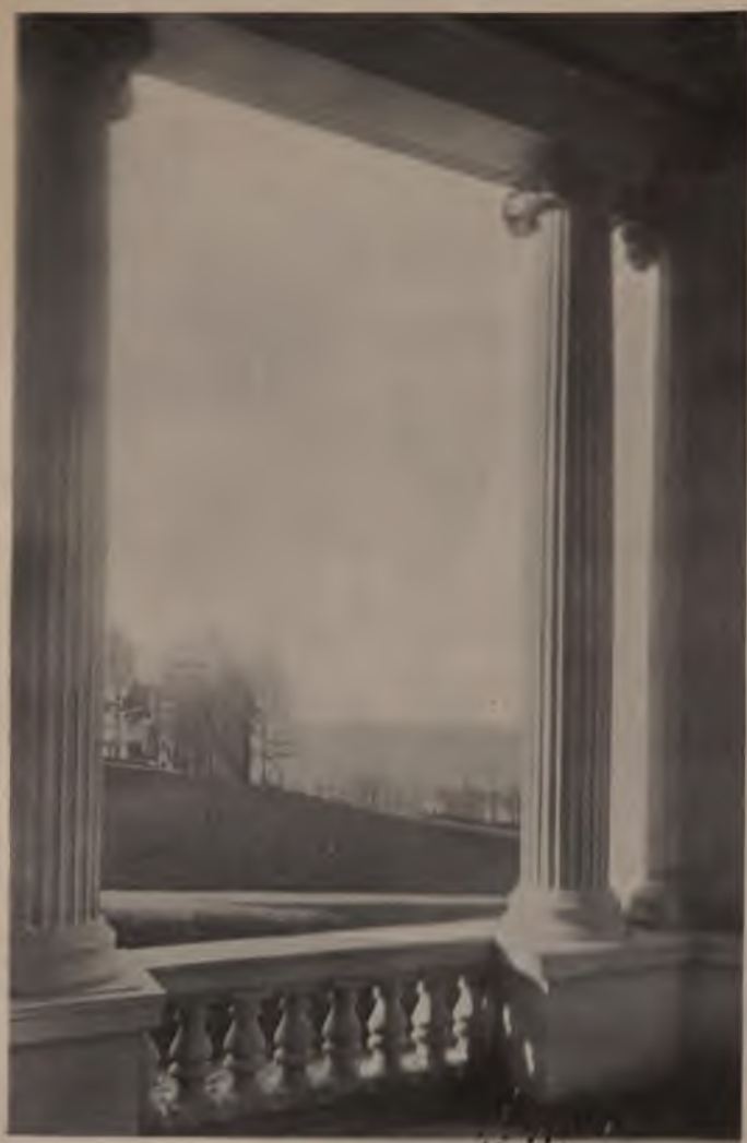
VIEW FROM AUTHORS' PAVILION LOOKING SOUTH
