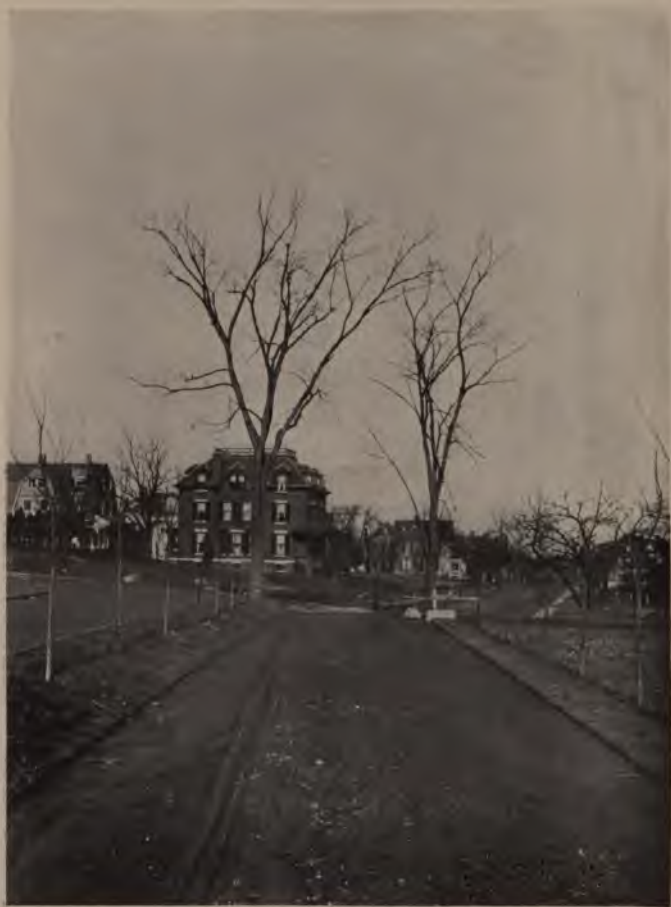
STUDENTS' ROAD LOOKING NORTH
