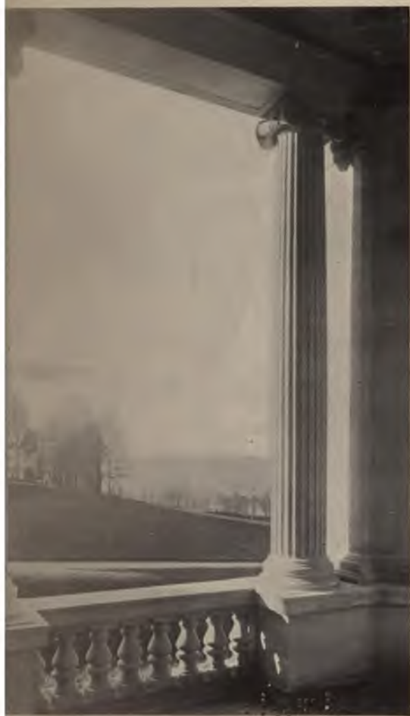
VIEW FROM AUTHORS' PAVILION LOOKING SOUTH
