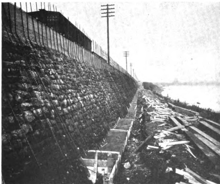
THE LEVEE WALL AT CAIRO, ILLINOIS In Process of Building
