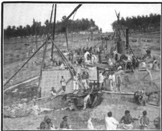
GERMANS BUILDING RAILWAY BRIDGE IN SHANTUNG
